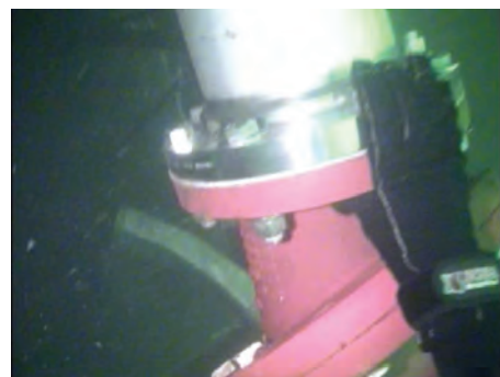
Replaced 8-inch Flange Gasket
