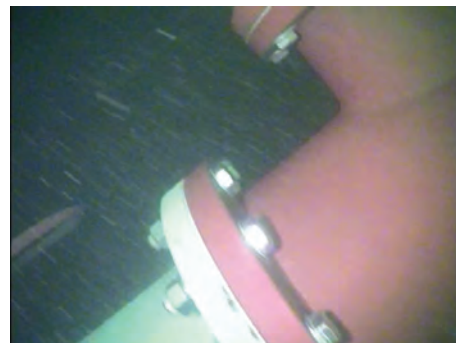
Replaced 14-inch Flange Gasket
