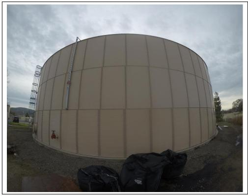
1.5MG Steel On-Grade Raw Water Tank
