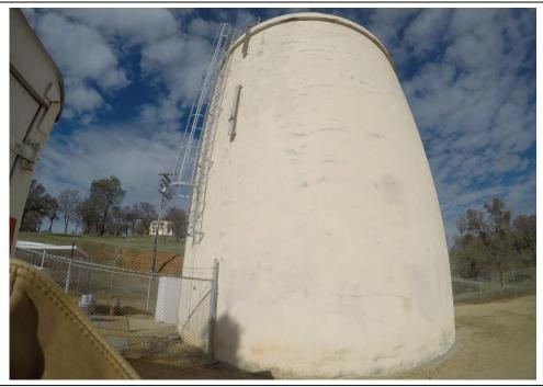
250KG Concrete On-Grade Enebro Tank
