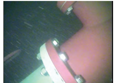
Replaced 14-inch Flange Gasket
