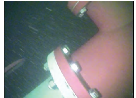
Replaced 14-inch Flange Gasket
