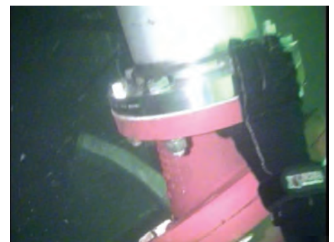
Replaced 8-inch Flange Gasket
