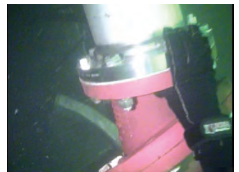
Replaced 8-inch Flange Gasket
